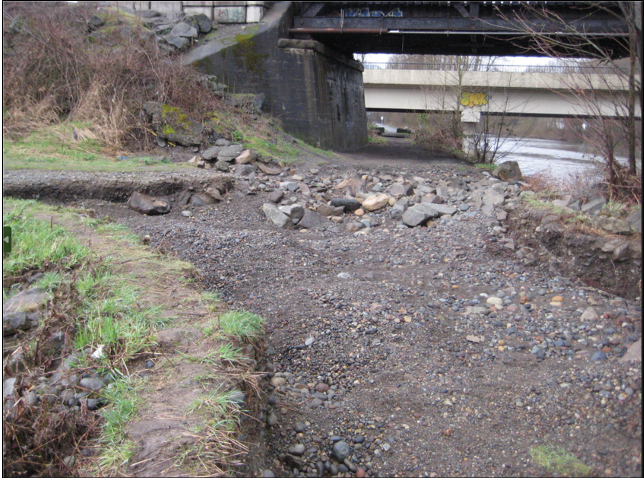
Figure 2.5: Scour and erosion of levee due to January 2009 flood at the location of the current outfall.
