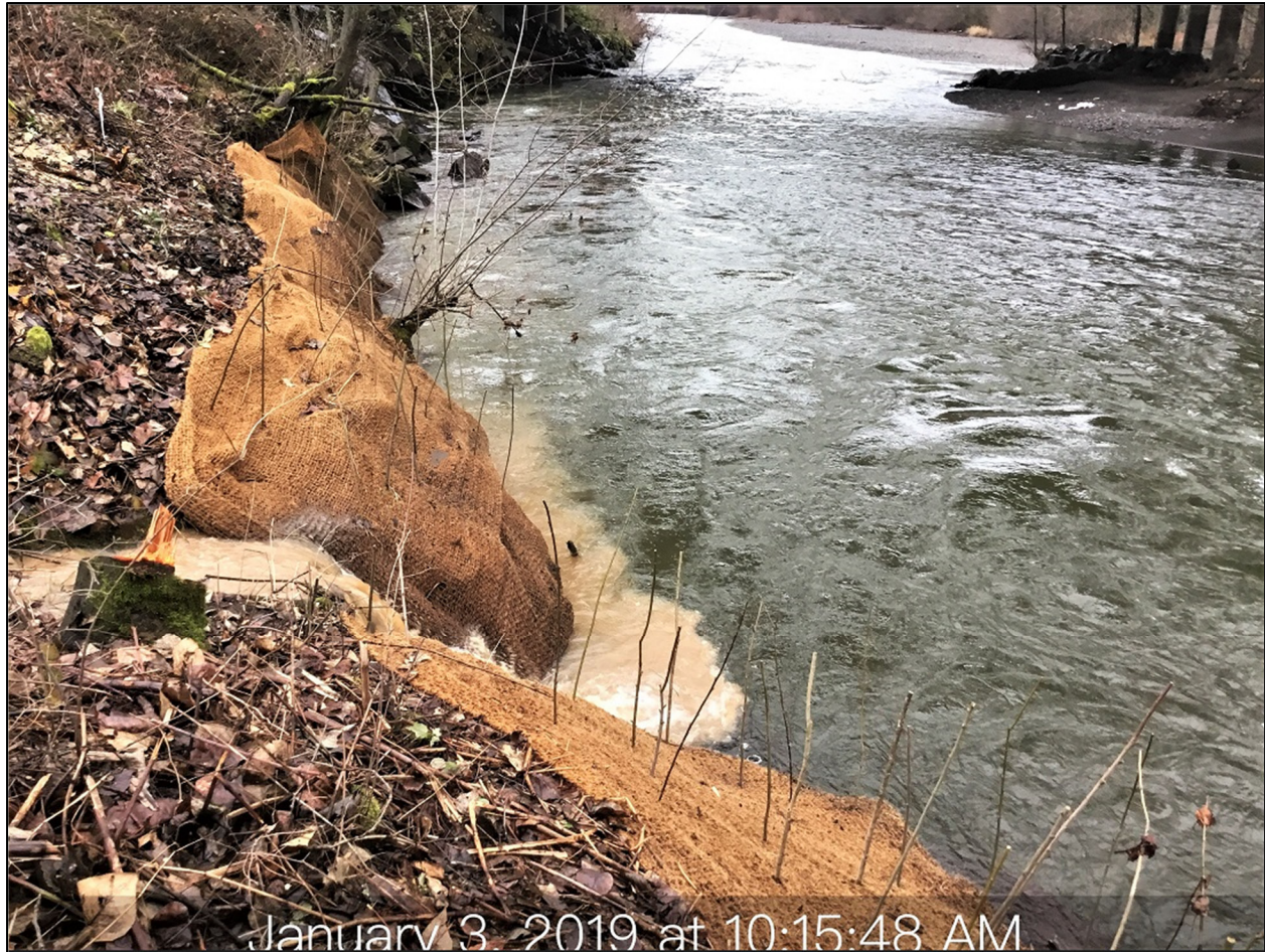
Figure 2.1: Initial coir installation, January 2019 or earlier. Note stormwater from pre-project outfall.
