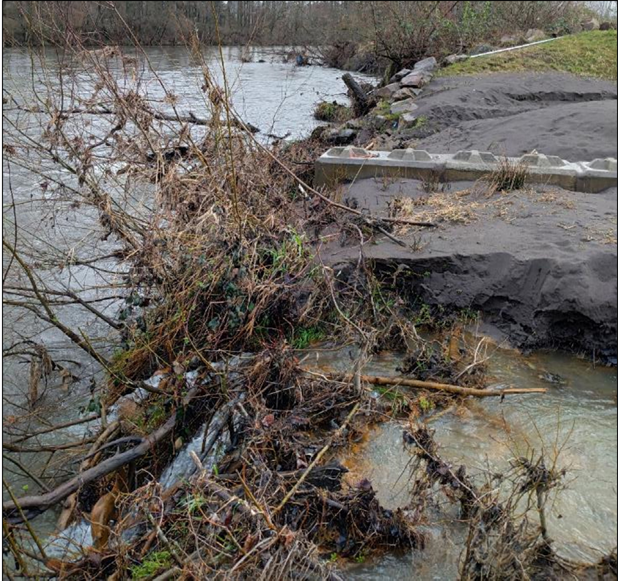
Figure 2.7: Concentrated flow spilling over, eroding, and undercutting vegetated bank. March 15, 2022, NHC.
